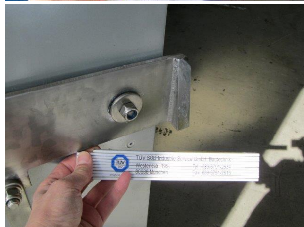
Fig. 5-4: Bolt mechanism and attachment screws on the protective door
